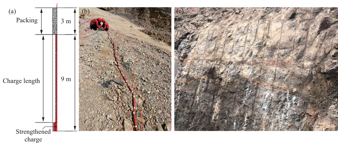
图 15 装药结构与现场爆后效果 Fig. 15 Charging structure and on-site post-explosion effect
